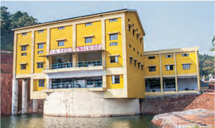
200 MLD Intake well and Pump House
