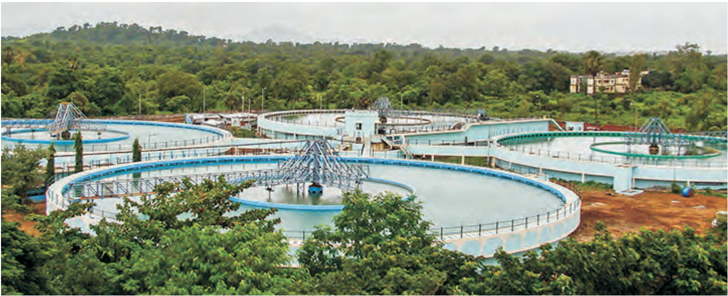
JNNURM TMC Project:180 MLD Clariflocculators
