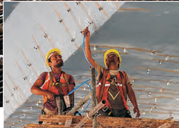
Epoxy Grouting
