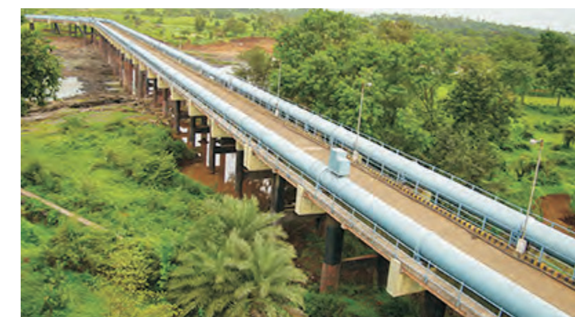
JNNURM Project: 1200 mm Dia. M.S. Raw Water Pumping Main
