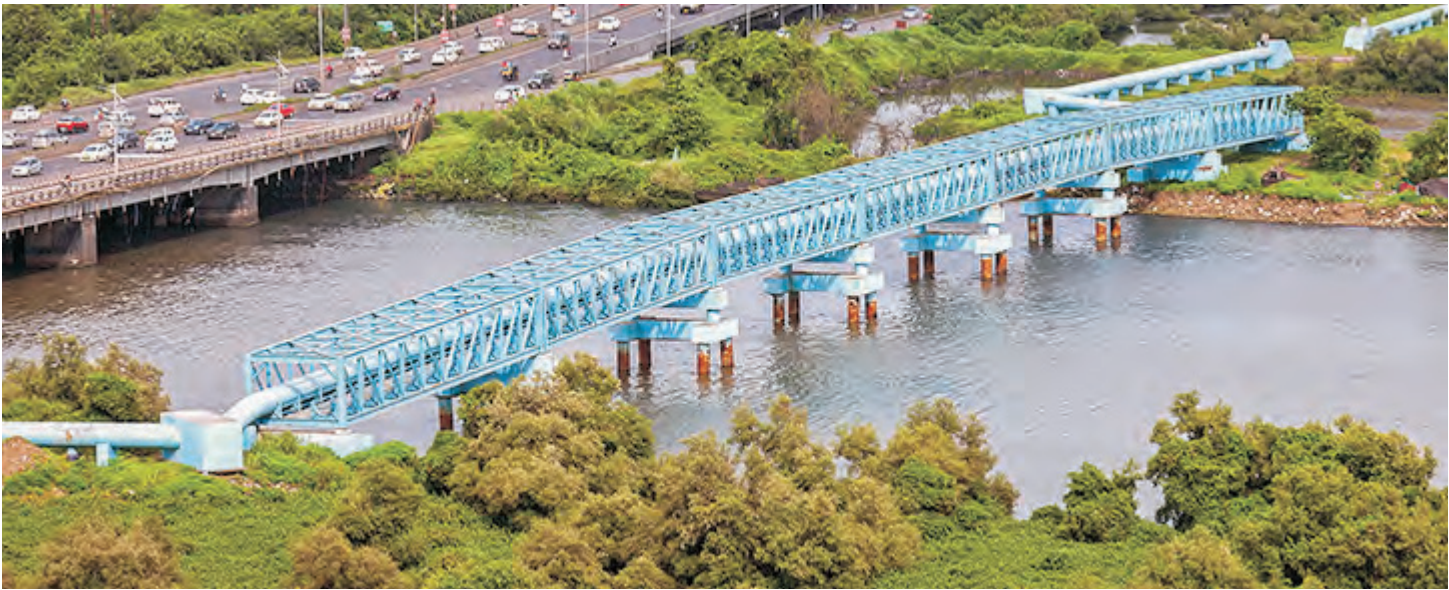
CIDCO: 1524 mm Dia M.S. Pipeline and structural Bridge over Taloja Creek
