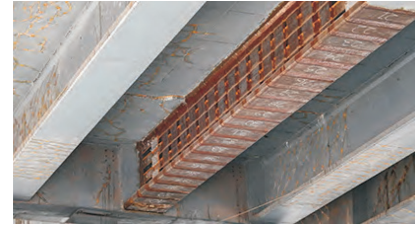
Fibre wrapping and prestressed carbon laminates
