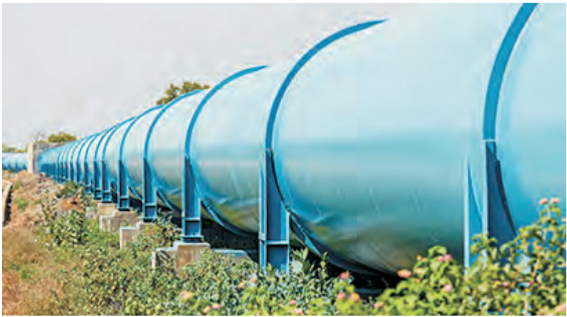
MCGM: 3000 mm Dia. Middle Vaitarna Water Pipeline
