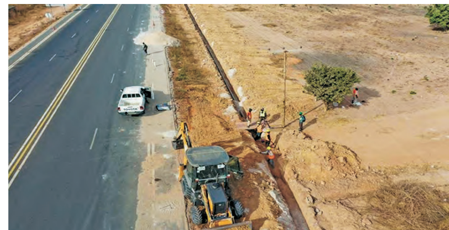
NAWEC: uPVC Pipe laying in Greater Banjul Area, Gambia
